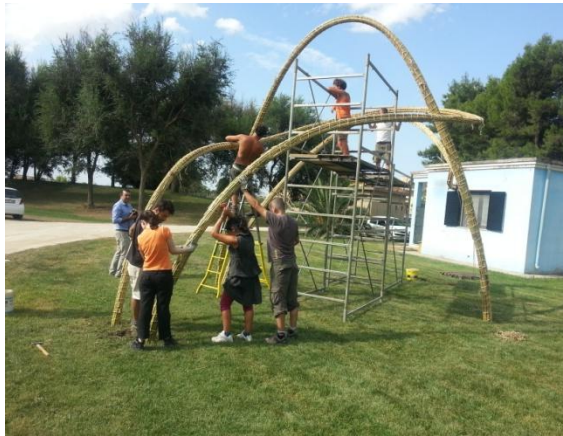
Εικόνα 8 Beyond Architecture Group and Laboratorio Architettura Naturali (LAN) organized a workshop to build a structure made of reeds and straw bales in Fiano Romano
