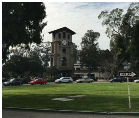
Figure 8 J. Morgan's reinforced concrete structure, El Campanil, a 72-foot (22 m) bell tower at Mills College (23)
