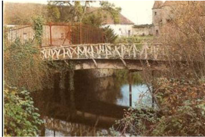
Figure 6 In 1873 Monier applied for an addition to patent 77165 to cover bridges, and in 1875 built his first bridge for the marquis de Tillière. It spans 14 metres across the moat of the chateau. (13)
