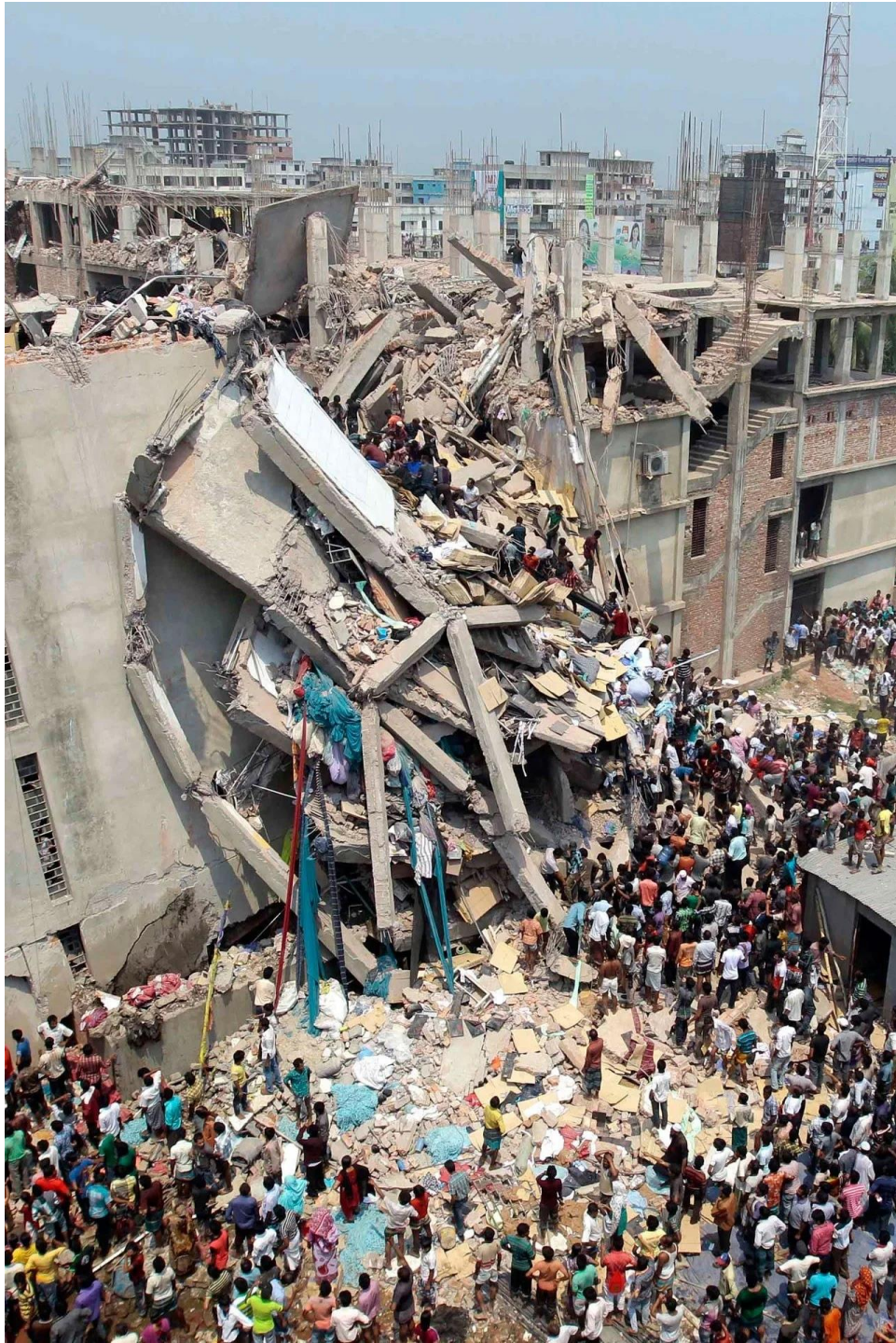
Figure 5 Bangladesh Factory Collapse Causes Garment Worker Fatalities, 2013, British Vogue
