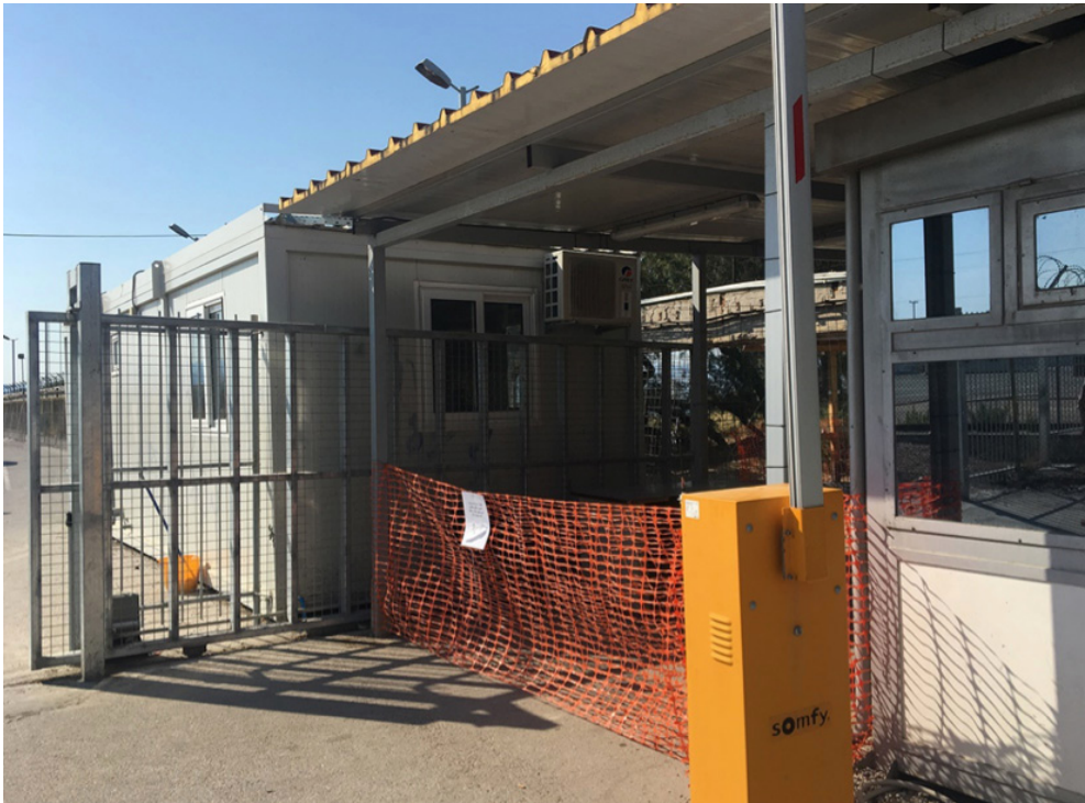
Figure 4. Skaramangkas Refugee Site entrance access point. A. Paraskevopoulou, 2017.
