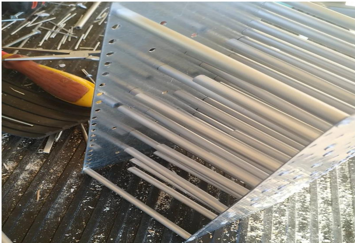
Installing the metal rods on the metal sheets for the instrument
